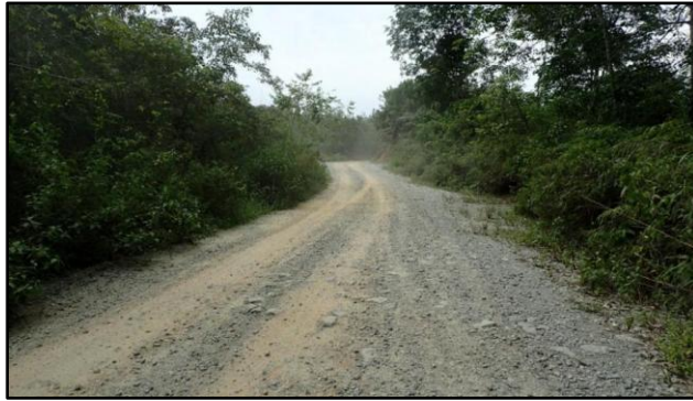
Plate 8.2.3: Example of Stabilized Access Road With Crusher Run to The Project Site
