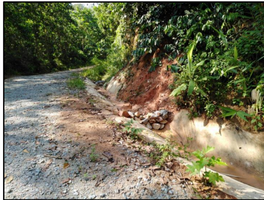
Plate 8.2.4: Example of Road Side Drain
