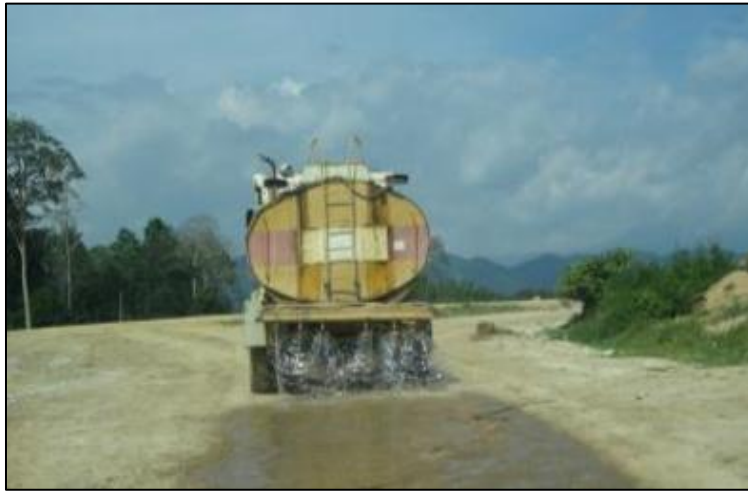
Plate 8.2.12: Example of Water Browser is used to reduce the dust pollution during construction
