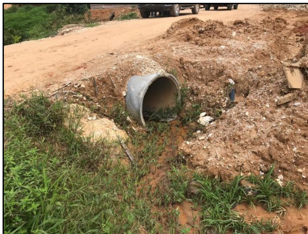
Plate 8.2.14: Example of Culvert
