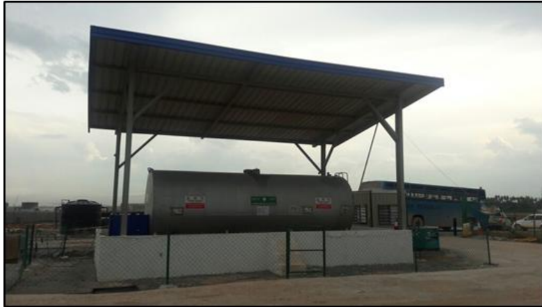
Plate 8.4.2: Example of Skid/Storage Tank on Stable Ground
