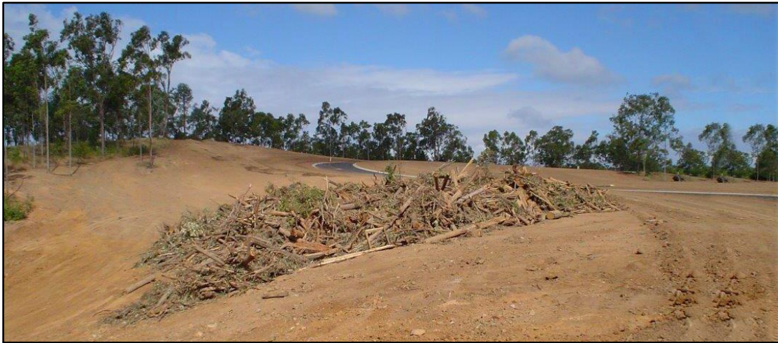
Plate 8.2.8: Mulching BMPs application locally in a land development project
