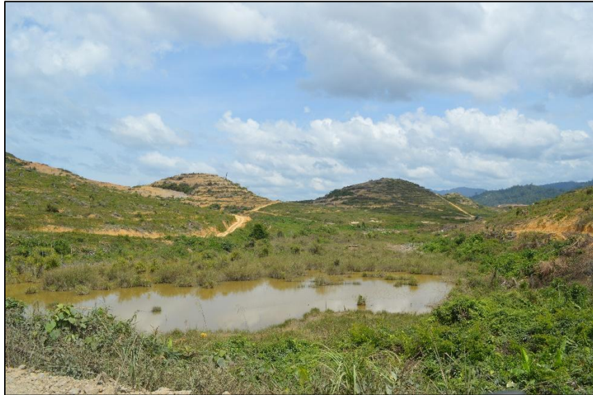
Plate 8.2.17 Example of Sediment basin at valley area
