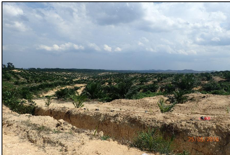
Plate 8.2.1 Example Perimeter Drain at the Project Site
